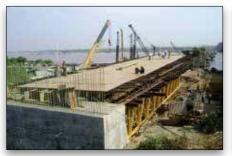
Figure 1: Superstructure Formwork Preparation
