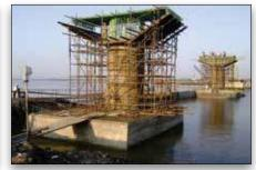
Figure 3: Preparing the Pier Cap Rebar Cage for Concrete Placement
