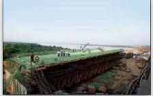
Figure 2: Preparing the Box Girder Rebar Cage for Concrete Placement
